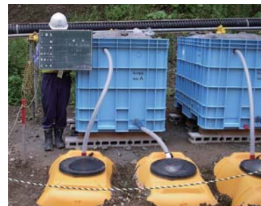
Soil-type rainwater exposure test in a cold district (at the filling treatment site along the Tozai Line on the city subway in Sendai City)
