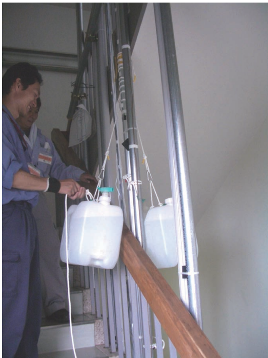
写真-1 ガイド管への錘の取り付け状況 Photo 1 Setting situation of the weight to a guide pipe.
