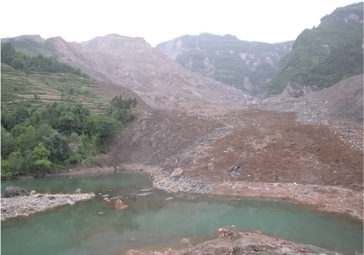
Photo. 4 Landslide and debris flow at Donghekou
