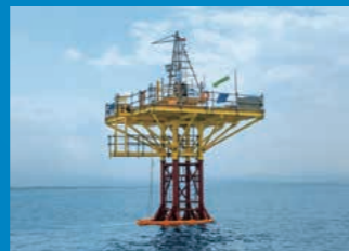
Offshore boring surveys
