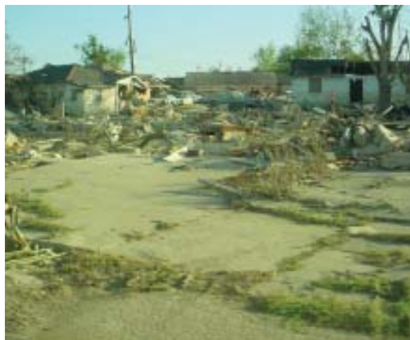
Damage in New Orleans from Hurricane Katrina
