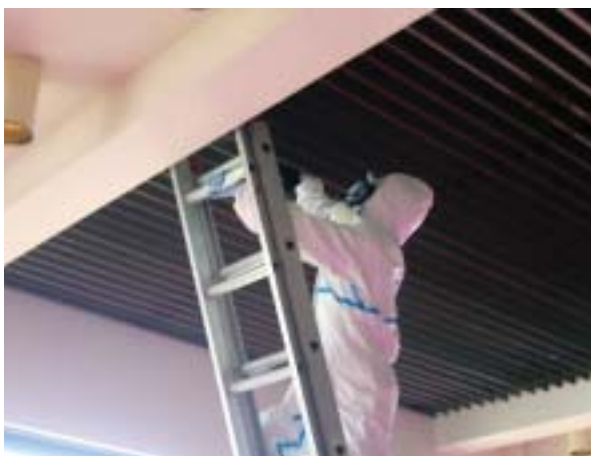
Inspection of Asbestos use
