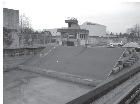
写真-2 模擬堤体の遠景 Photo 2 View of the river dike model.
