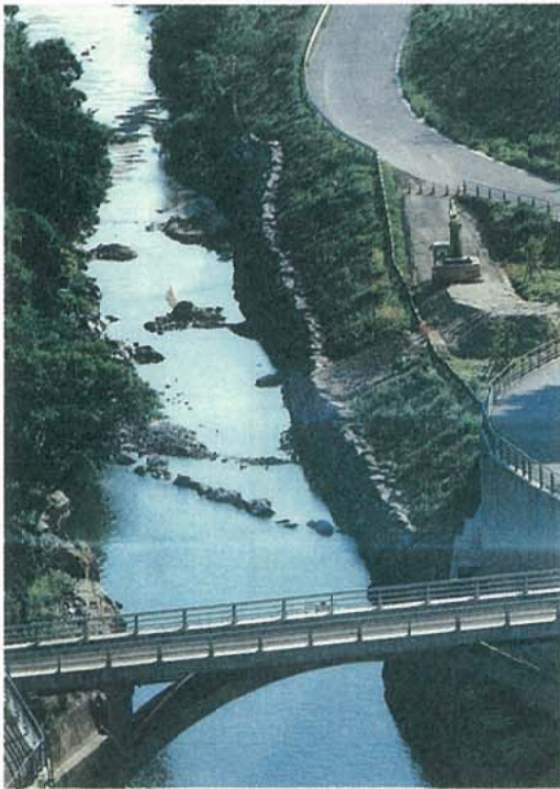
写真-2 放流後の土砂設置箇所 Photo.2 Installed sediment downstream after draw-off experiment
