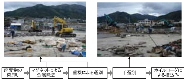
図-4 1次選別（粗選別）の手順例 Fig. 4 Example procedures for primary separation (Rough separation)
